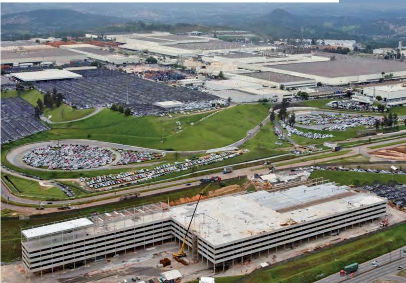
Betim - MG - BRASILE Citta' di Betim, deposito logistico multipiano FIAT, cinque livelli City of Betim, FIAT multilevel logistic depot, five floor level
